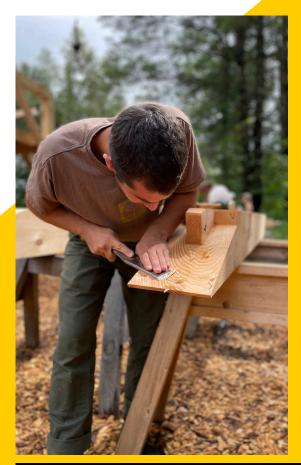
In the summer of 2023, Yestermorrow students embarked on timber framing journey to construct our friend Eddie Merma's home. Over the span of a couple of weeks, these two classes learned the techniques and methods necessary to raise a timber frame structure.
